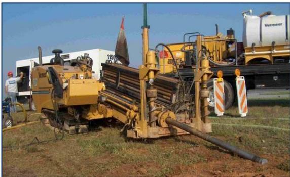
Once the directional drilling is complete, Kalin will install the remainder of the water main, including replacement of the services to your home. Please note that water main installation will involve work on the west side of the roadway. The Kalin's crew will retain existing pavement on the west side of the roadway as long as possible, but there will come a time when this pavement must be removed.
